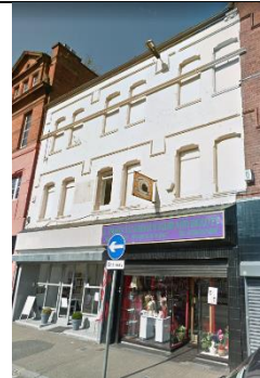
29A-31 NORTH STREET (ST. ANNE'S BUILDINGS)
