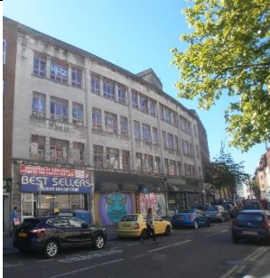
12-22 NORTH STREET (CANADA HOUSE)
