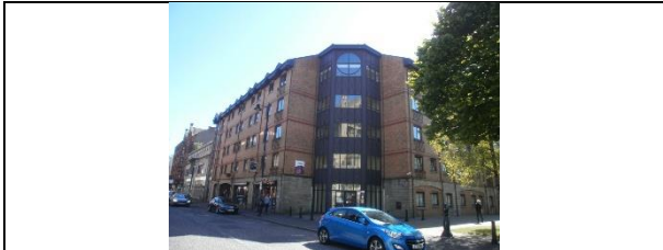
32-40 DONEGALL STREET (SHAC HOUSING)
