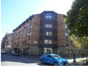
32-40 DONEGALL STREET (SHAC HOUSING)
